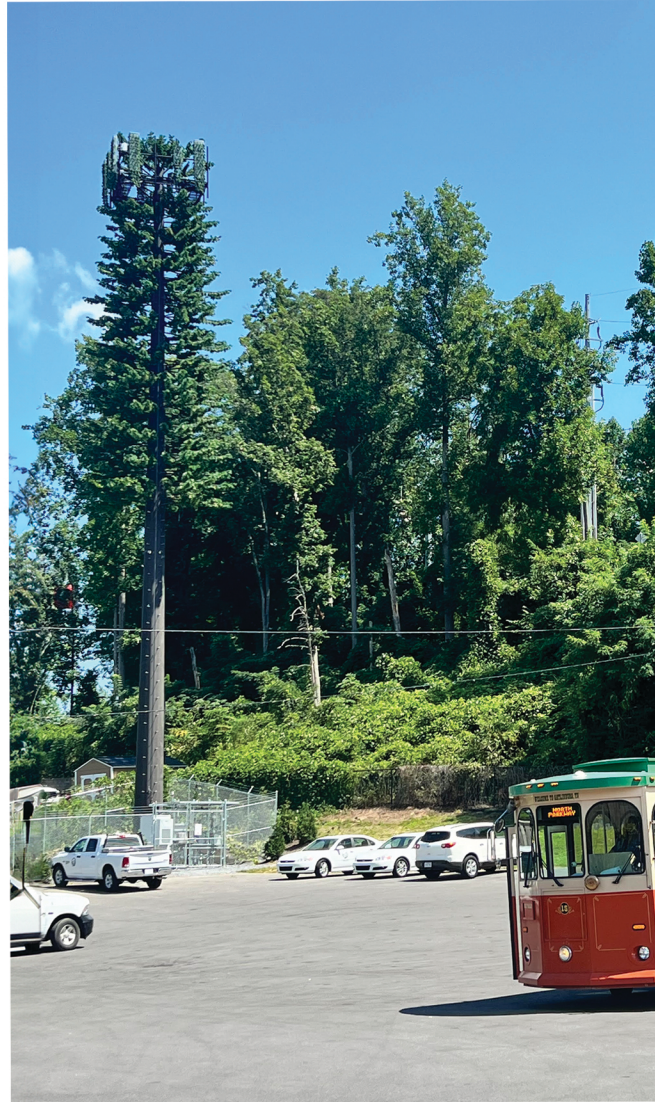
120' Monopine Gatlinburg Elementary School
